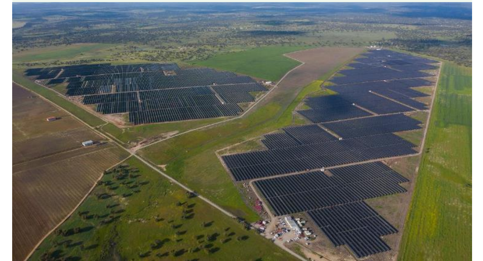
100MW photovoltaic project in Spain
